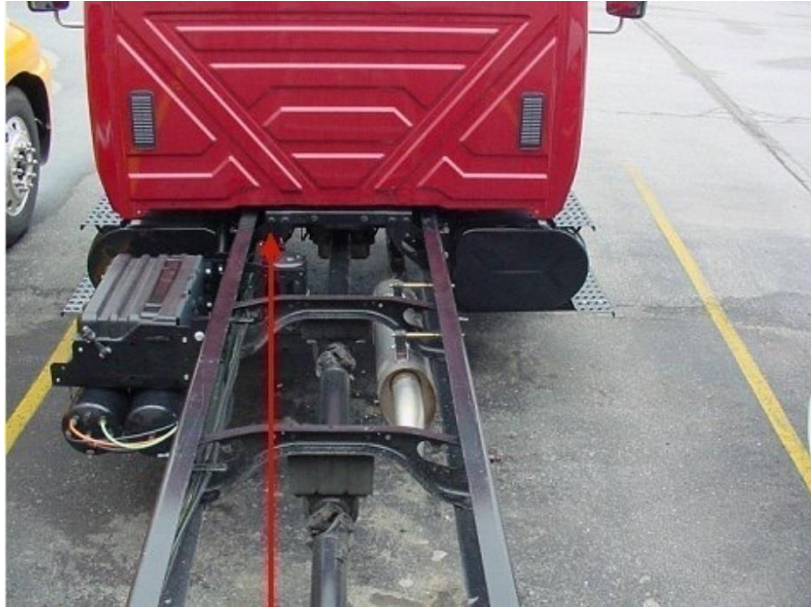
Arrow Indicates Location of Work Light Connector (Straight Truck)
